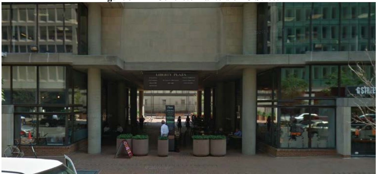
Figure 3-2 Concrete Planters on G Street
