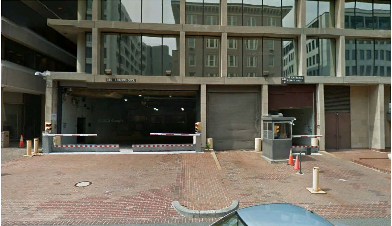
Figure 3-5 Raised Vehicular Plate Barriers at Loading Dock Entrance on F Street
