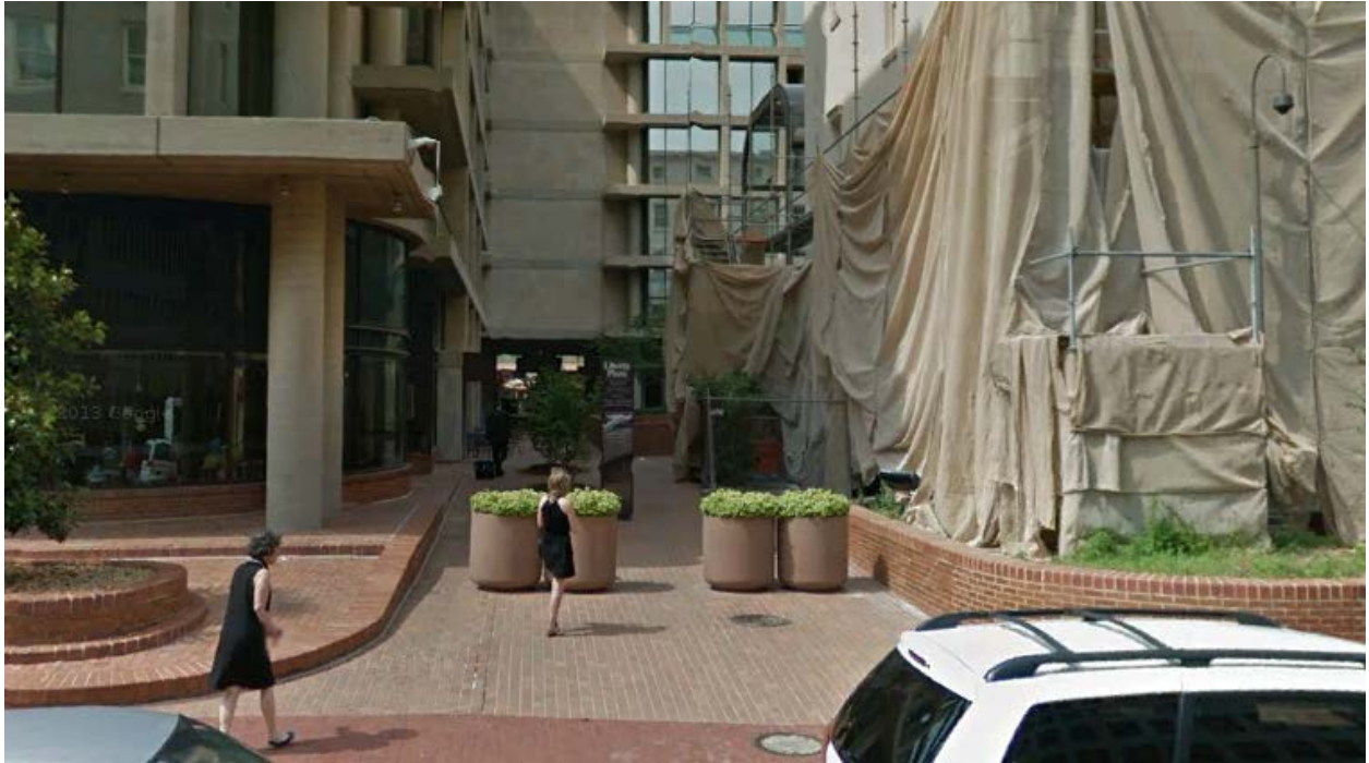
Figure 3-3 Concrete Planters on F Street
