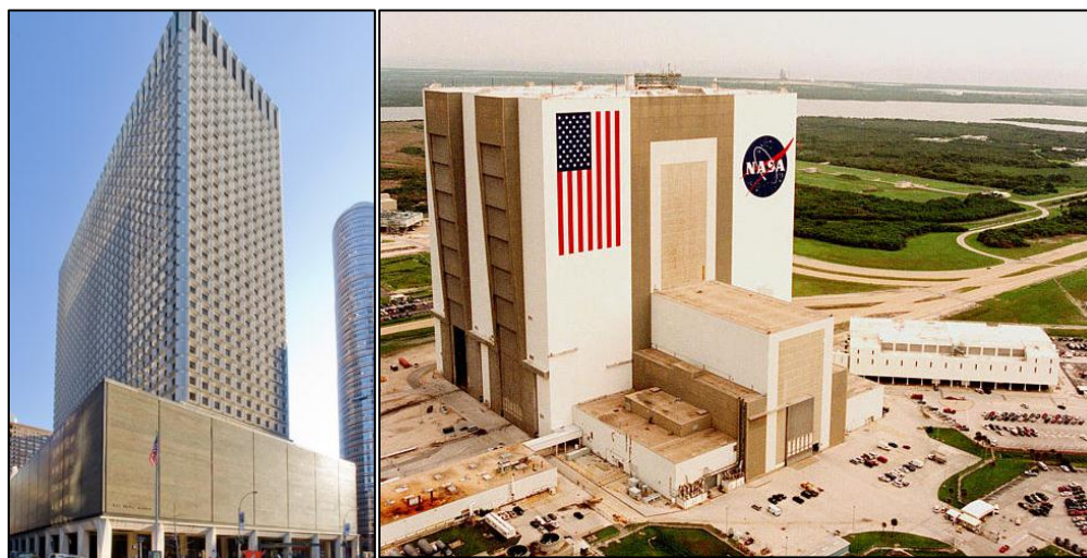
Figure 18: Max Urbahn Associates-Designed Buildings 909 Third Street in New York City (Left) and the NASA Vehicle Assembly Building (Right) (NASA 1999; Vornado Realty Trust 2013).
