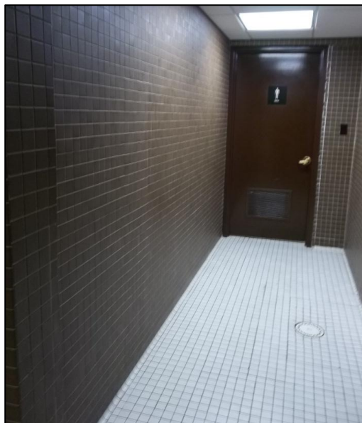
Figure 12: View of the Use of Tiles In and Around the Bathrooms.
