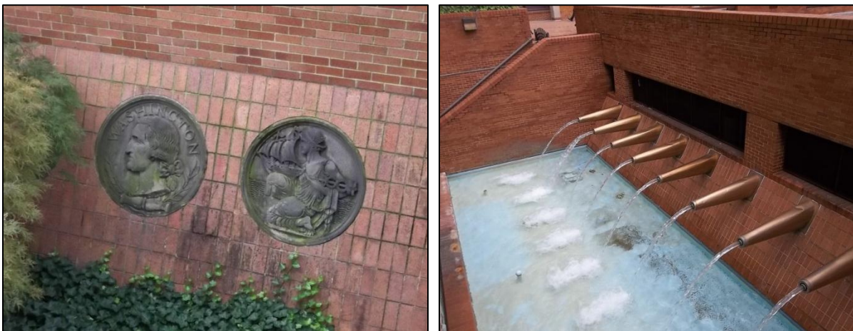
Figure 17: Two of the Four Bronze Medallions on the Eastern Plaza Wall (Left) and the Water Feature on the West Side of Plaza (Right).
