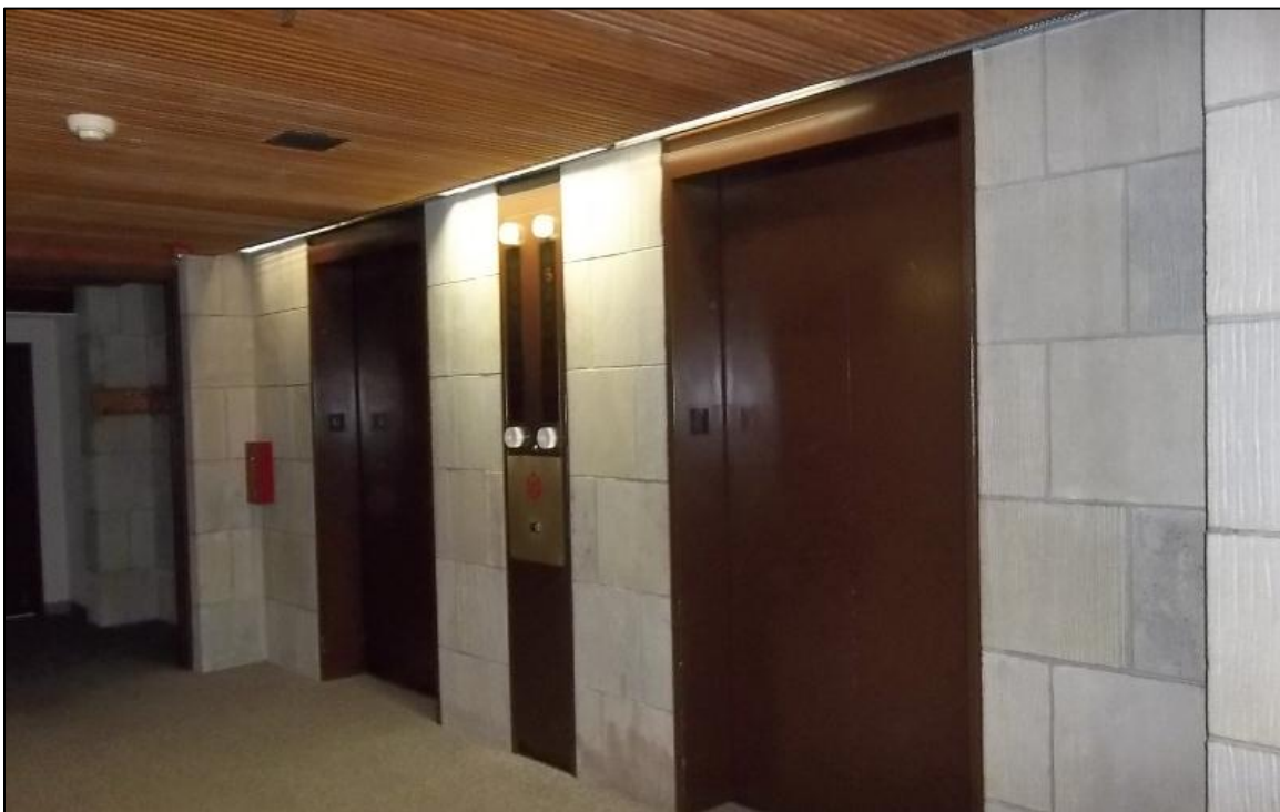
Figure 8: Detail of the Original Elevator Elements and Limestone Blocks.
