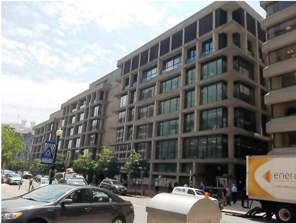
North Elevation of 1700 G Street, NW (The Federal Home Loan Bank Board Building).
