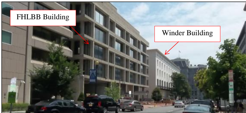
Figure 19: Looking East Along F Street, NW Toward 17 th Street. Note how the horizontal elements of the FHLBB building are similar to those of the Winder Building.
