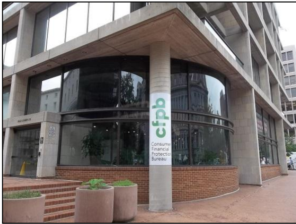
Figure 30: Curved Glass on Southeast-corner Windows.
