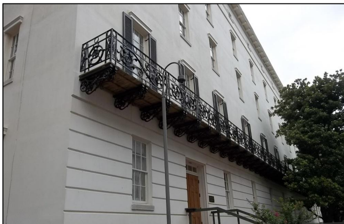
Figure 24: Restored Balcony on the South Elevation of the Winder Building.
