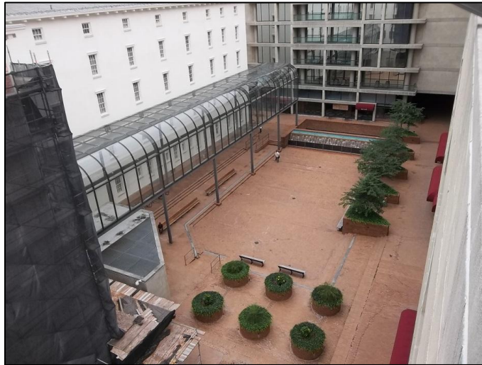
Figure 15: Looking Southwest at Liberty Plaza. Note the triangular and circular planters.
