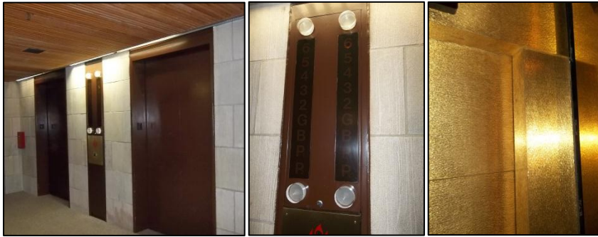
Figure 39: Original Elevators and Elevator Features.
