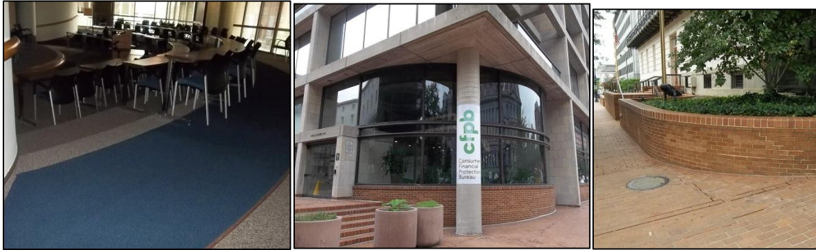
Figure 29: Use of Curvilinear Elements Throughout the Building and Site: Built-in Concrete Steps in Current Auditorium, Southeast-Corner Windows, and Brick Planters in Plaza.
