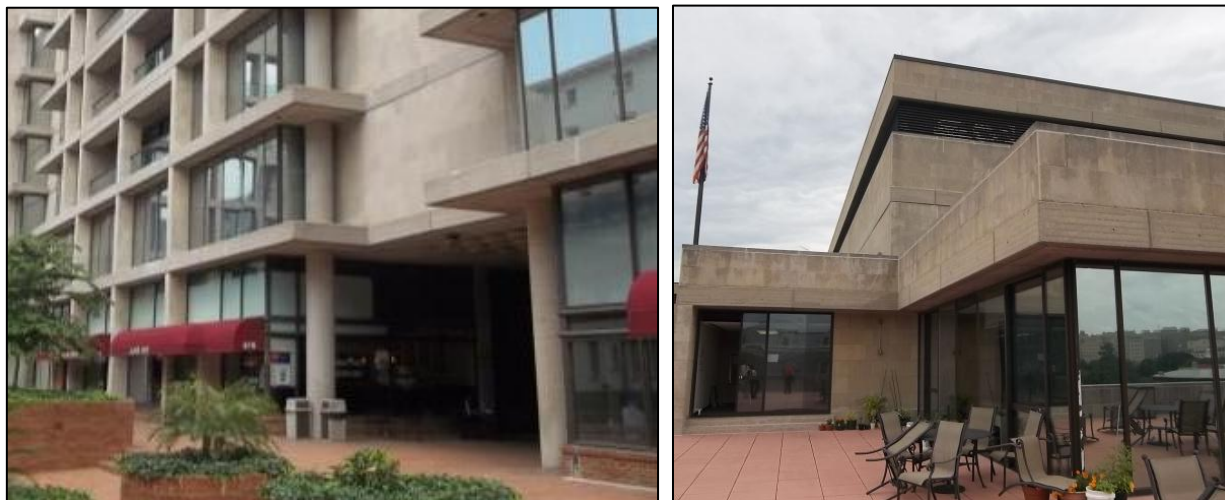
Figure 4: Ground Level of the FHLBB Building (left) and Sixth Floor Veranda (Right).
