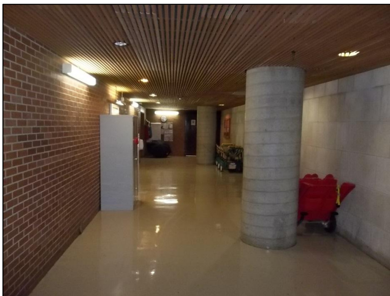
Figure 13: Overview of the Basement.
