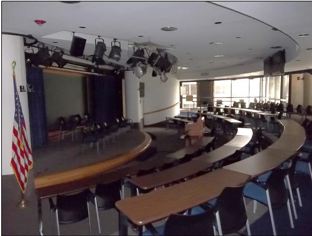
Figure 10: Auditorium on the Second Floor, Looking North.
