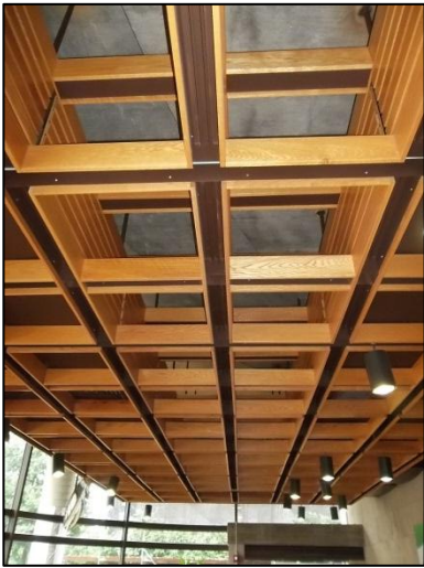
Figure 52: Wood, Coffered Ceiling in Lobby.
